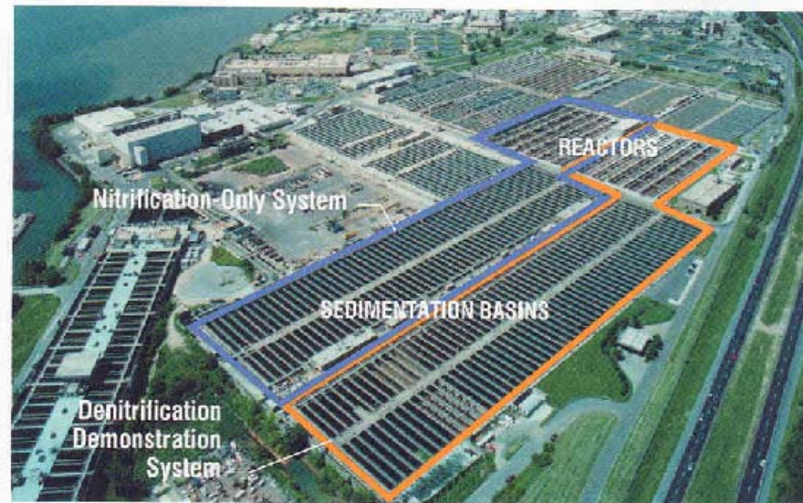
Denitrification demonstration reactors and sedimentation basins at the Blue Plains Facility are outlined in orange. The control basin is outlined in blue.
